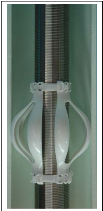
Stainless supplied by DEPS with a Kwik-ZIP centralizer in PVC bore-casing ready for the sand to be pored in to create the gravel pack
